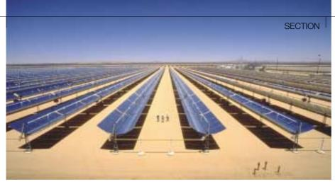
Figure 4 Parabolic trough concentrating solar collector field of the 150 MW (5  $\times$  30 MW) steam cycle solar electricity generating systems at Kramer Junction, California (Source: KJC)
