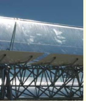
Enhanced parabolic trough structure of the EUROTOUGH project facility at Plataforma Solar de Almeria, Spain
