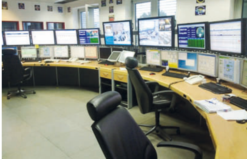
Fig. 2-7 Ground Operations Control Room (GoCR)
