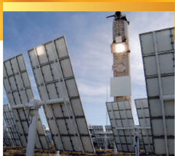
The solar hybrid gas turbine test plant
