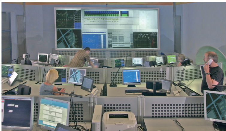
The ACCES control room featuring 10 operator working positions and a high resolution display wall
