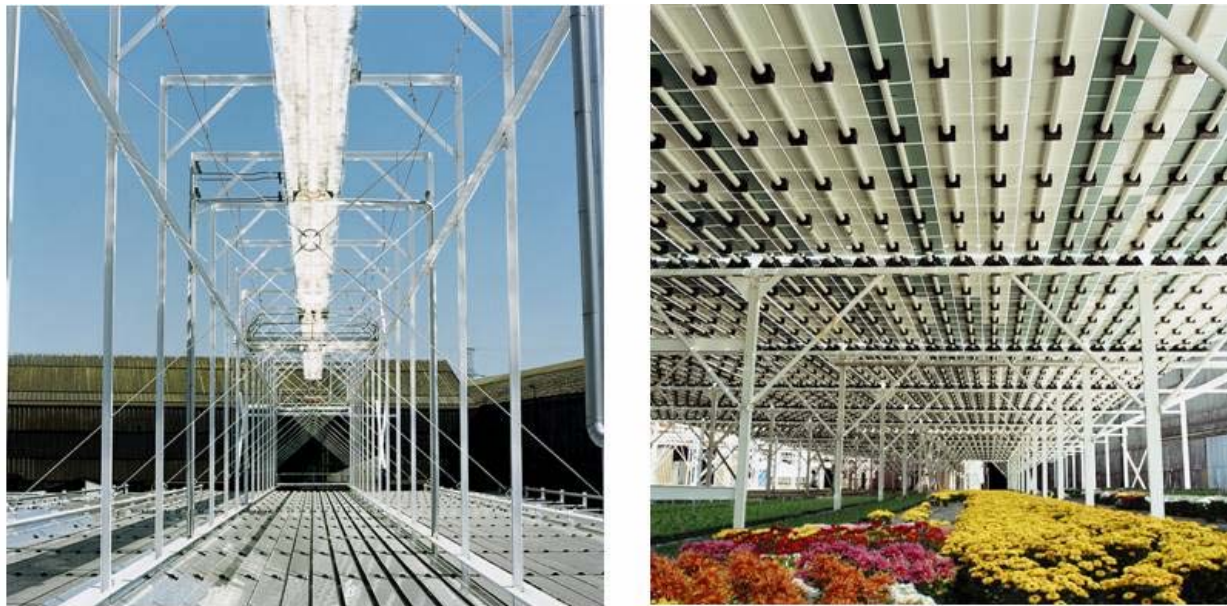
Figure 5-19: Photo of the top of a Linear Fresnel Concentrating Solar Collector and artist view of a greenhouse installed underneath to protect the plants from excessive irradiance and evaporation. This could be a concept for multi-purpose plants for power, water and horticulture. Other local uses include shade for parking and the production of steam for cooling and process heat. (Source: Solarmundo, DLR)
