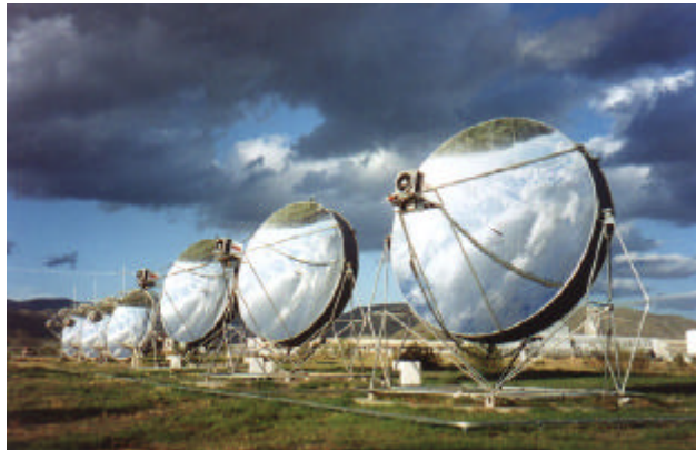
Fig. 14 The six DISTAL systems at the Plataforma Solar de Almería in Spain.
