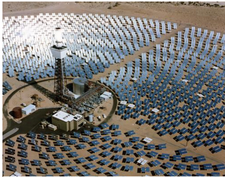
Fig. 8 Solar Two, a molten salt receiver in the USA
