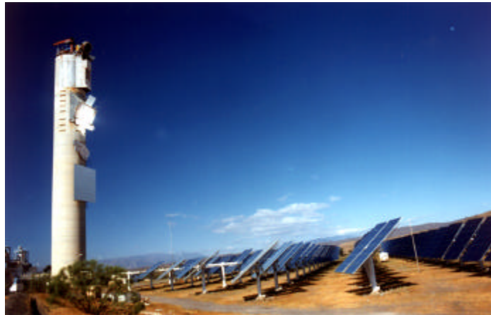
Fig. 9 The CESA I test facility at the Plataforma Solar de Almería in Spain
