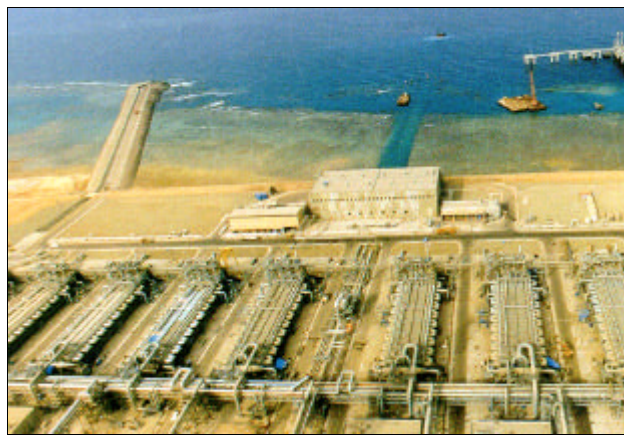
Fig. 13: Makkah-Taif Multi-Stage-Flash Desalination Plant with 223,000 m 3 /day Capacity (Source: Mitsubishi Heavy Industries Ltd.)
