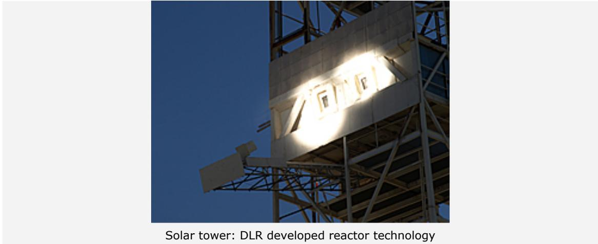
Renewable hydrogen production using solar energy and the resulting storage of solar energy by this chemical energy carrier are of the greatest technological and economic interest for the energy industry. After an extensive thermal qualification of the solar tower plant, which took place this summer, the plant was recently fitted for the first time with solar absorbers covered in a special coating that enables them to split water and thus to produce hydrogen in a CO2-free way.
