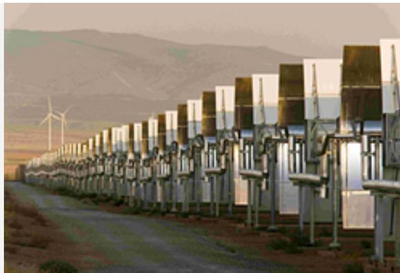
Parabolic troughs are constantly directed to face the sun
