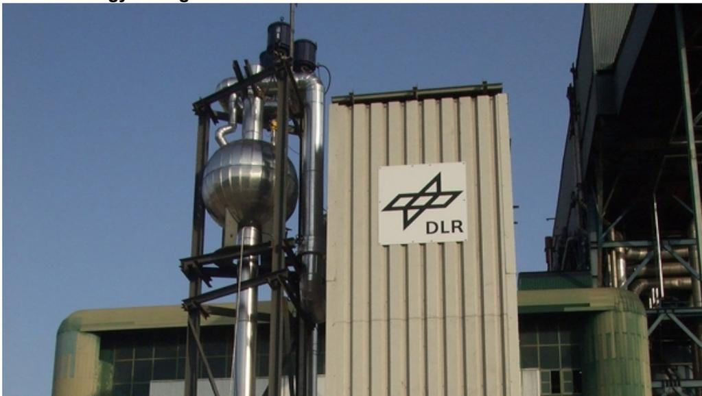
The salt-based latent heat storage system works using a phase transition. At 305 degrees Celsius, the salt absorbs energy by transitioning from a solid to a liquid state. Latent heat is 'hidden' energy. Energy is accumulated as the storage medium changes phase from solid to liquid.
