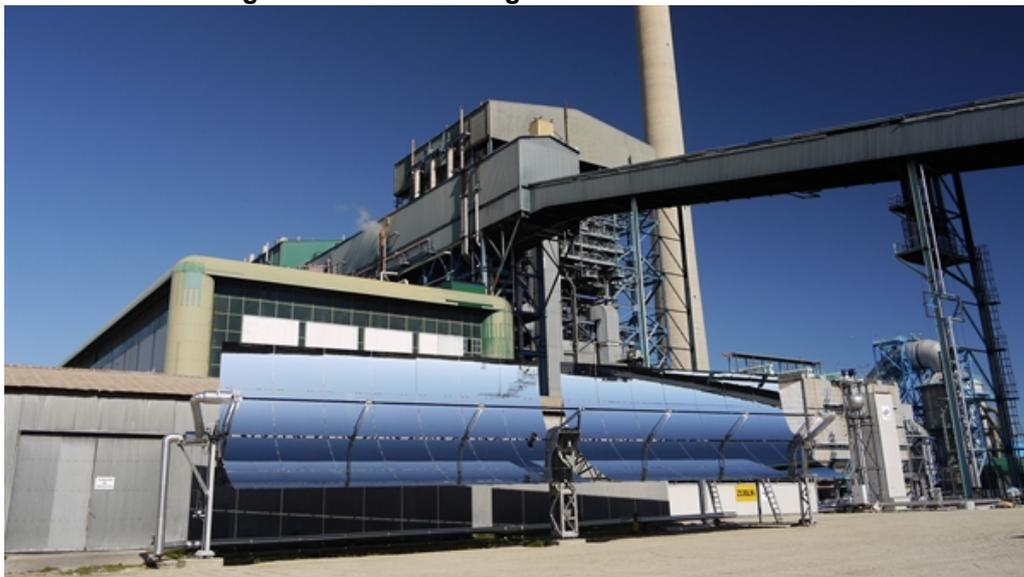
The German Aerospace Center (DLR) and Endesa test direct solar steam generation and energy storage in this pilot plant in Carboneras, located in southern Spain. In this type of solar
