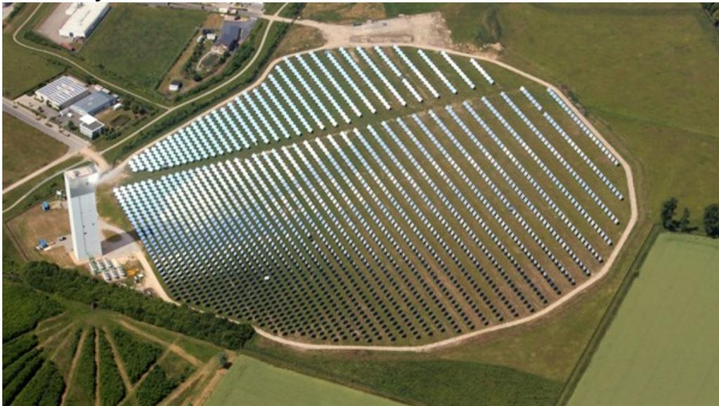
Sunlight is reflected off over 2000 mirrors onto the high-temperature receiver of the power plant tower in Jülich. In a solar power plant, solar radiation is converted into heat in the receiver.
