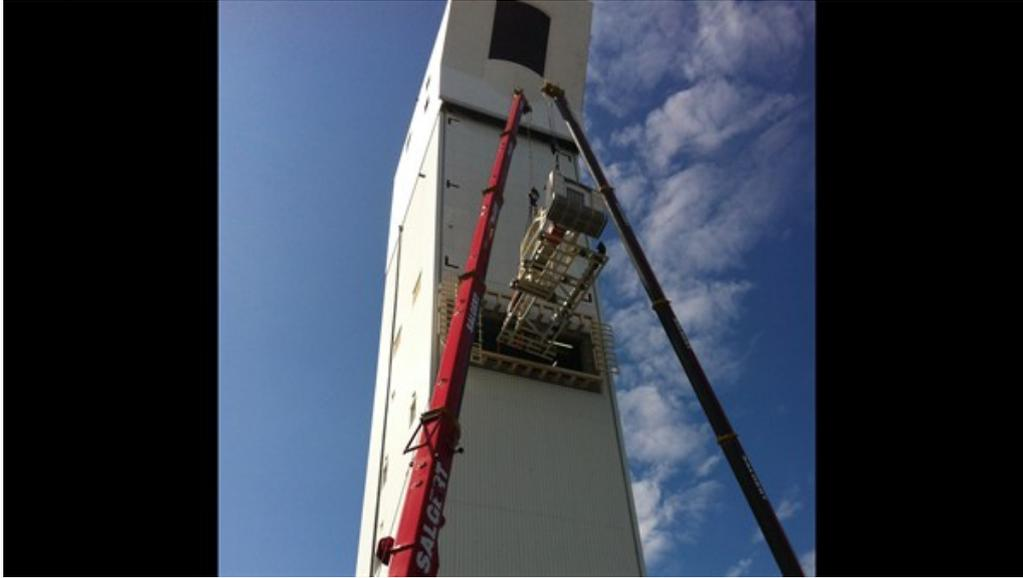
The new test receiver is installed at the research level of the DLR solar tower in Jülich Using two cranes. The test receiver on the research level is easily accessible to the scientists. The research level makes it easy modify the test receiver and allows the use of extensive metrology to accurately monitor its operation.
