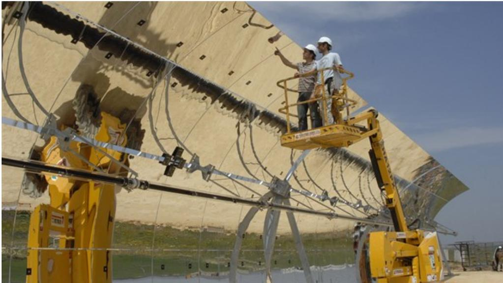
Marc Röger and his team are measuring the parabolic mirrors and adjusting them so they are in an optimal position.
