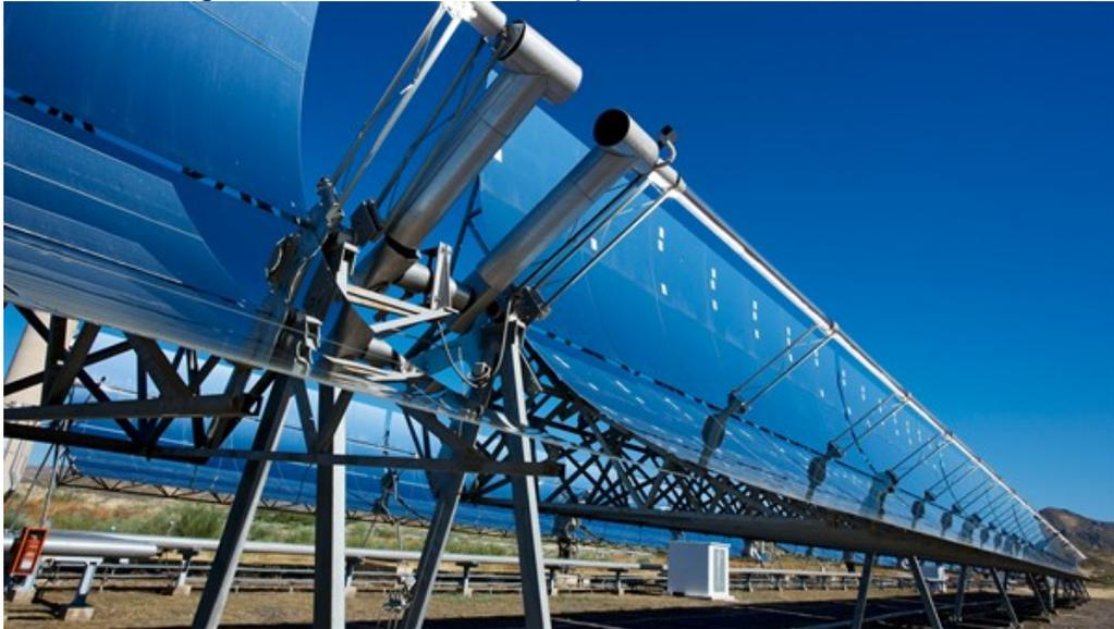
The simulation program FreeGreenius calculates profitability and the optimal design of a power plant. The picture shows a parabolic trough collector at the Plataforma Solar de Almería (PSA) in southern Spain.
