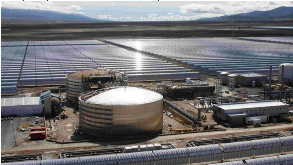
In the background, the parabolic trough power plant is visible. The solar power plant 'Andasol 1' is equipped with 600 parabolic trough collectors that provide the thermal energy to operate the generators. In the foreground is the salt-based energy storage facility.
