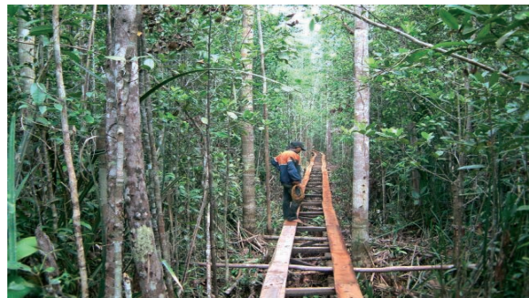
Figure 2.64 A 15 km long wooden bridge installed for collecting ground measurements in the Mawas Peat forest test site (Kalimantan, Indonesia, 2004).
