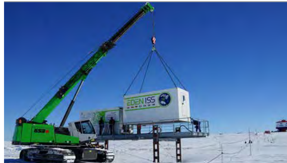
Assisted by F. LAEISZ and the AWI on-site construction team, the two research containers were removed from the raised platform
