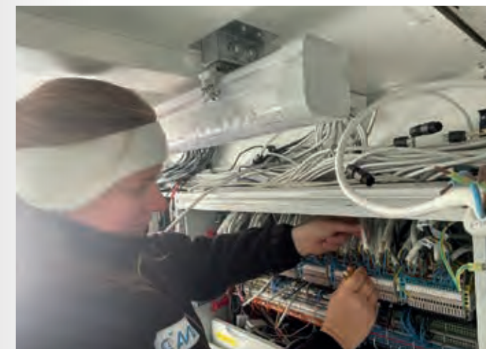
Claudia Philpot disconnects the power and data lines to the FEG equipments
