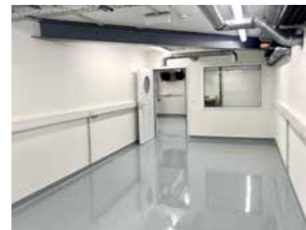
Multi-purpose lab area prior to outfitting
