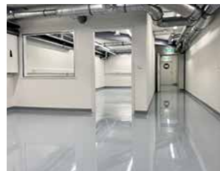
CEA control room prior to outfitting
