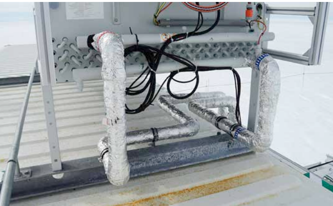
Insulated thermal piping connecting to the free cooler on top of the MTF
