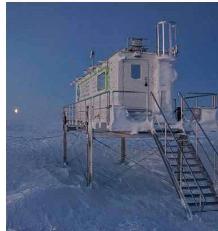
Snow and ice build-up around the EDEN ISS MTF
