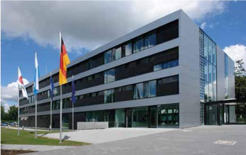
The EOC building in Oberpfaffenhofen
