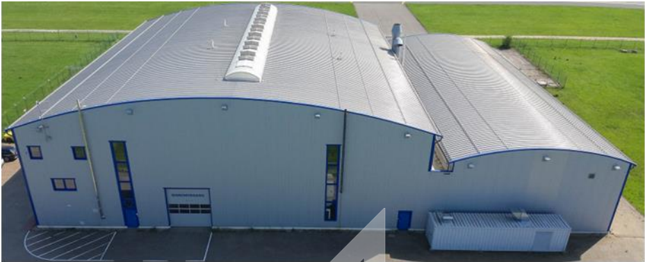
UAS hangar, workshop, charging center
