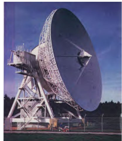
Figure 1-37: A 34-m Cassegrain dish antenna of DLR.
