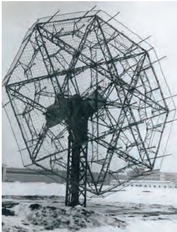
Figure 1-34: The test monopulse tracking antenna in Oberpfaffenhofen (diameter 11 m).
