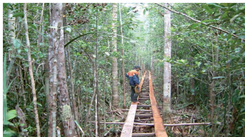
Figure 3-13: INDREX II: A 15 km-long wooden bridge installed for collecting ground measurements in the Mawas peat forest test site (Kalimantan, Indonesia, 2004).
