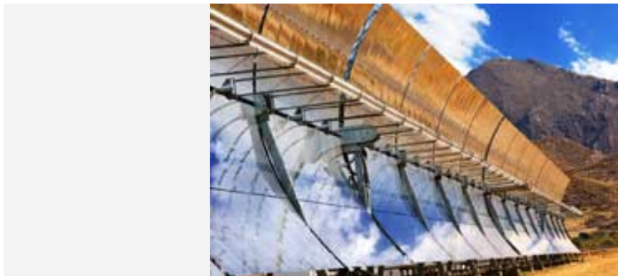
Parabolic trough concentrator on Solar de Almería platform
