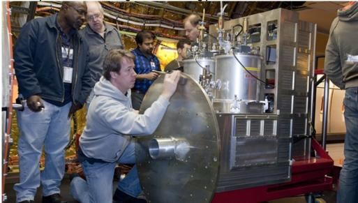
Final inspection and cleaning of the mounting plate before mating with the telescope. Rainer Strecker (DSI quality Management) works with the mounting plate: Alvin Mitchell and Rolf Güsten are in the background.
