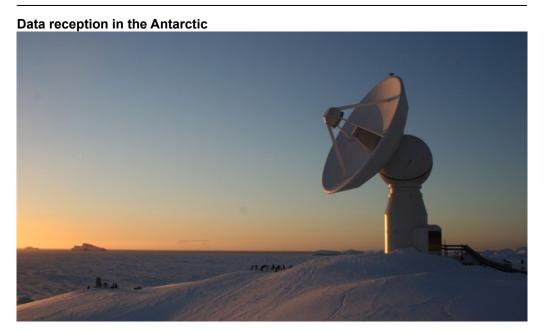
The O'Higgins German Antarctic Receiving Station (GARS) was established in 1991. Since then, the nine-metre antenna has been receiving satellite data – even in extremely stormy conditions.
