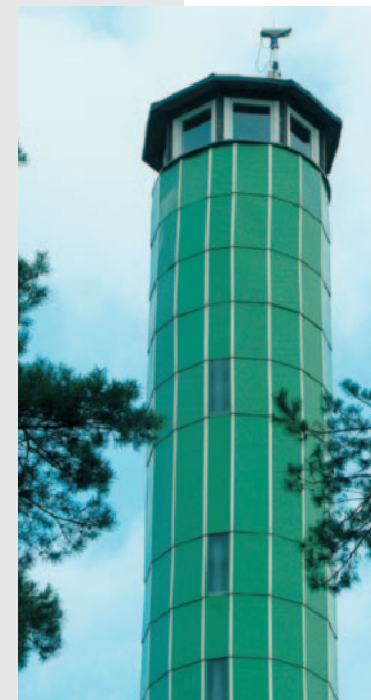
Working with IQ Wireless GmbH, DLR has developed the 'Fire-Watch' system, which employs technology derived from space-based optical sensor systems. FireWatch detects forest fires in their early stages by automatically recognising smoke, even at night. The image shows the FireWatch technology on the fire lookout tower at Zesch am See, about 45 kilometres south of Berlin.
