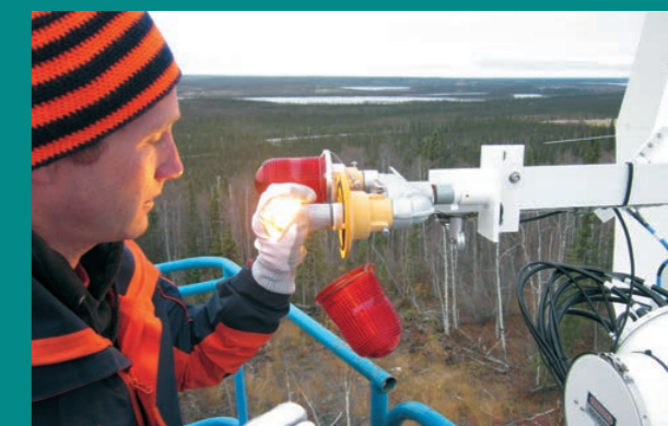
Part of the maintenance – replacing lamps on the antenna.
