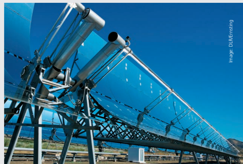
The simulation program FreeGreenius calculates profitability and the optimal design of a power plant. This image shows a parabolic trough collector at the Plataforma Solar de Almería (PSA) in southern Spain.
