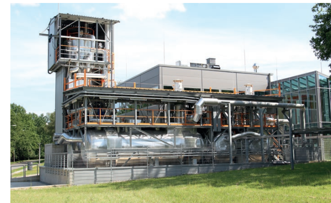
Research for the Energy Transition: High-temperature heat storage materials are key for controllable, renewable electricity. At the DLR test facility TESIS, companies can test components to be used in molten salt storage.
