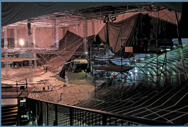
The sculpture was assembled bit by bit from aluminium girders, a structure of iron bars and panels, and lifted up by heavy duty engines. The screen for the animations of the DLR Earth Observation Center measures over 2000 square metres.
