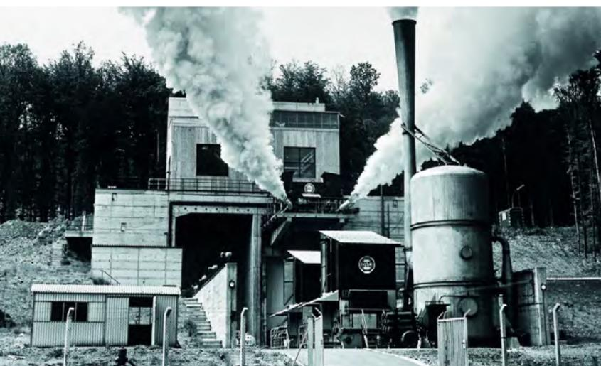
From 1966, the Astris upper stage engine was tested under high-altitude conditions on the P4 test stand. The site engineers developed special steam generators for the operation of the high-altitude system. Since the 1970s, the P4 stand has been retrofitted several times for the Ariane programme. Today, Ariane's Aestus and Vinci upper-stage engines are tested there.
