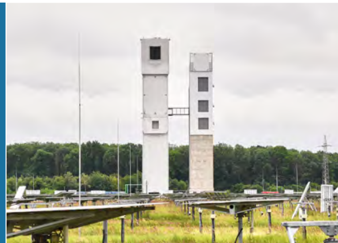
At DLR's Jülich site, the Institute operates a solar thermal tower power plant (left). Since 2020, the site is also home to the Multifocus Tower (right), in which new solar technologies can be tested.
