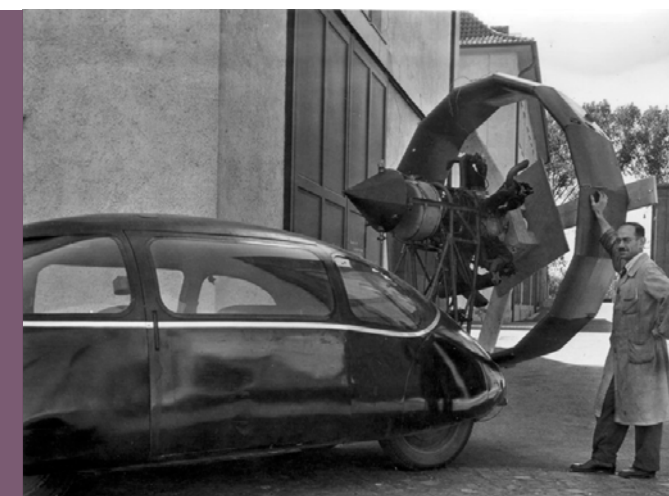
Engineer Karl Schlör developed the AVA experimental car in 1938. In 1942, he brought a captured Russian propeller to AVA and mounted it on the car for test purposes.
