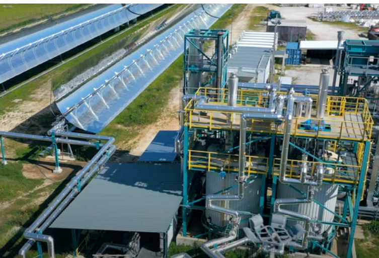
At the Évora Molten Salt Platform in Portugal, DLR is working with the University of Évora to research how molten salt can be used as a heat transfer medium in solar thermal power plants. Until now, oil has been used as the heat transfer medium in such power plants.
