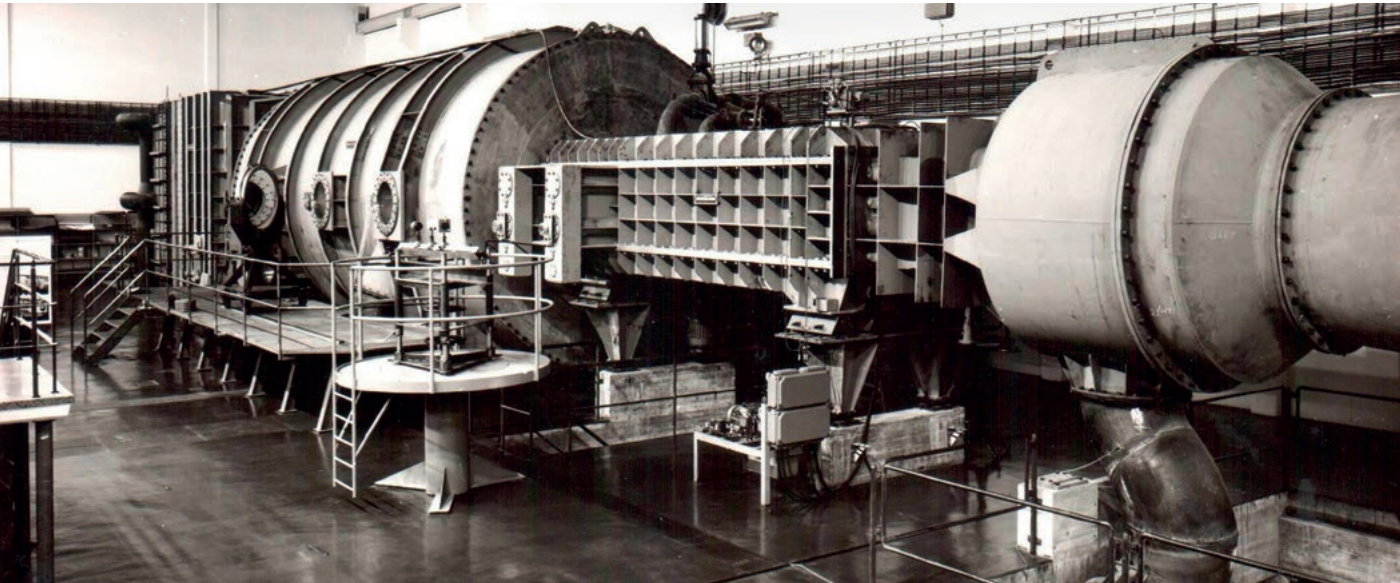
Wind tunnels often remain in use for a surprisingly long time. They need to be repeatedly modernised, as has been the case with the Transonic Wind Tunnel in Göttingen, which has been refitted several times since its construction in 1963.
