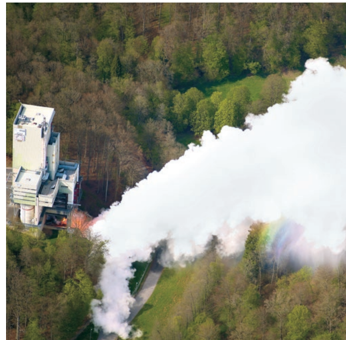
Aerial image of a Vulcain 2 test on the P5 test stand at DLR Lampoldshausen
