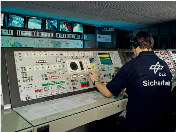
DLR safety engineers monitoring the large-scale test at the safety panel in the control room of the test stands
