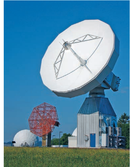
The 13-metre antenna requires outstanding manufacturing precision and motion accuracy. The parabolic reflector is manufactured to a tolerance of one tenth of a millimetre and can withstand external temperatures of all seasons.
