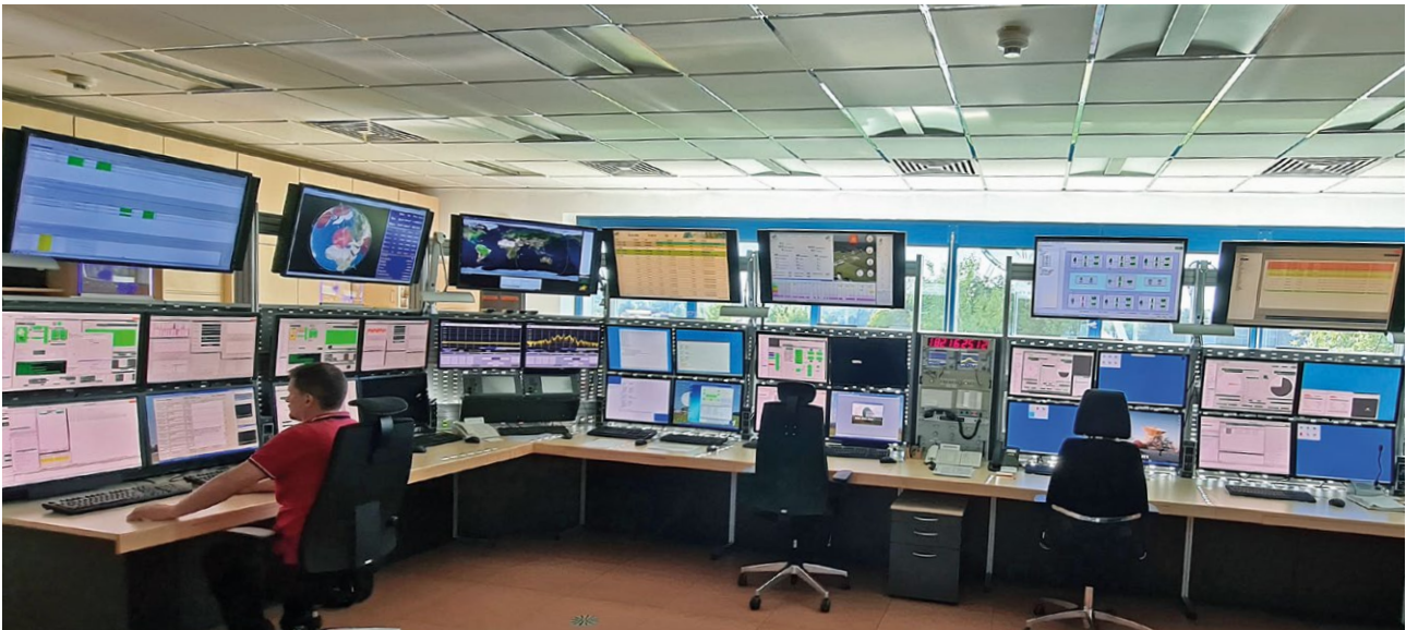
Fig. 4-3 Ground Station antenna control room
