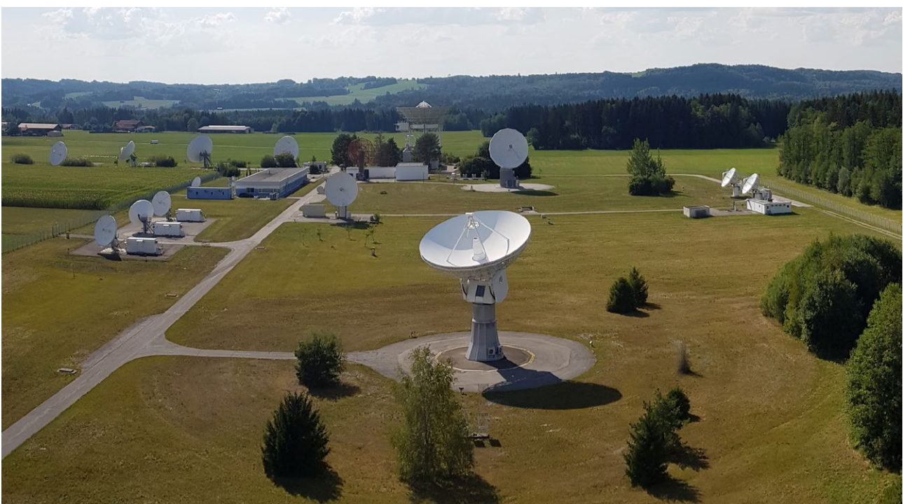
Fig. 5-3 The 15m II S/X-band antenna in Weilheim
