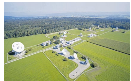
Fig. 2-3 Ground Station located at Weilheim
