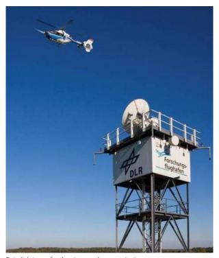
Data link tower for the air-ground communication
