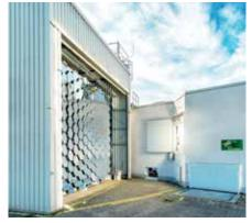
The DLR solar furnace: the mirrors of the concentrator focus the radiation onto an experimental set-up inside the laboratory building
