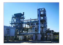
Power: 1.8 MWth @ 14.0 MPa / 560 °C Economizer/evaporator, air cooled condenser, pressure reducing station
