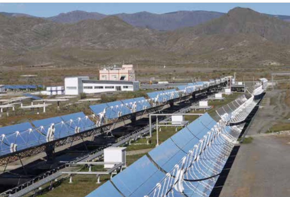
Figure 1: DISS test loop at PSA upgraded to once-through operation at 120 bar/500°C.
