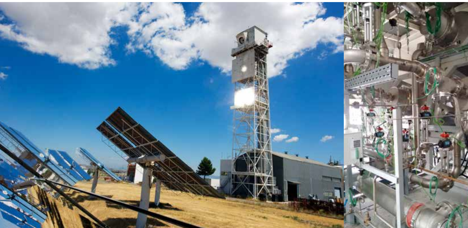
Figure 2: Solar tower (left) at PSA hosting the 750 kW demonstration plant (right) for solar thermochemical hydrogen production. Picture left: DLR/Lannert.
