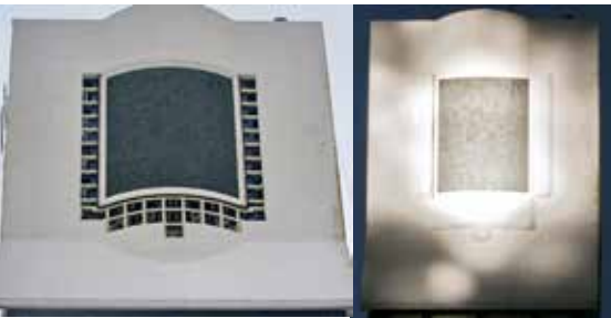
Installation of receiver return air nozzles (left) and solar test after completion (right), 2015.
