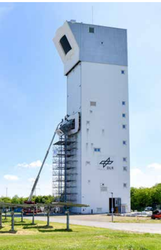
Mounting of the particle receiver CentRec® at the Jülich Solar Tower's research level in May 2017.
