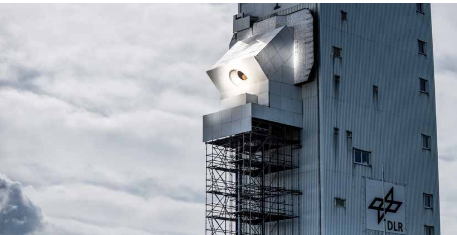
Figure 2: CentRec® Receiver prototype during on-sun operation in DLR's Jülich Solar Tower.
