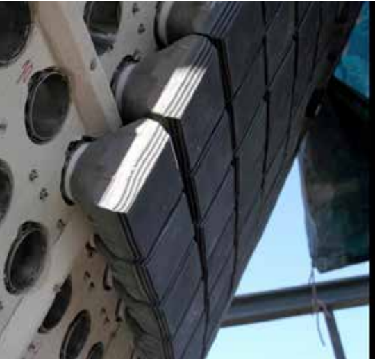
Figure 1: Ceramic absorber modules in the HiTRec receiver support structure.
