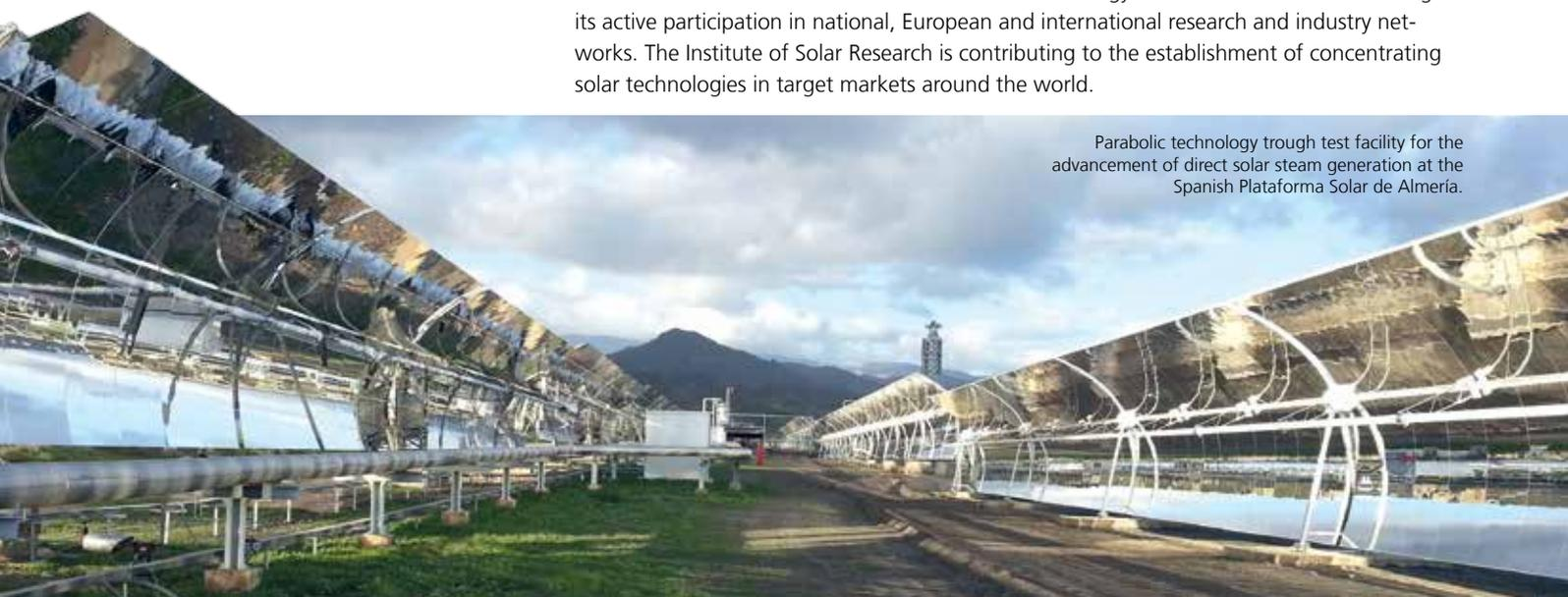
Parabolic technology trough test facility for the advancement of direct solar steam generation at the Spanish Plataforma Solar de Almería.
