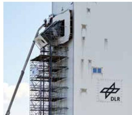
Installation of the CentRec particle receiver on the 'Research Level' of the Juelich Solar Tower.
