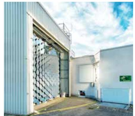
The DLR solar furnace: the mirrors of the concentrator focus the radiation onto an experimental set-up inside the laboratory building.
