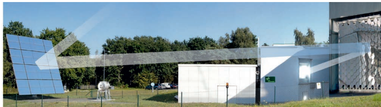
Beam path of the High-flux solar furnace (fotomontage)
