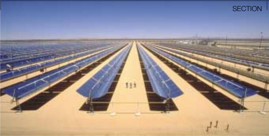
**Figure 4** Parabolic trough concentrating solar collector field of the 150 MW (5 × 30 MW) steam cycle solar electricity generating systems at Kramer Junction, California (Source: KJC)
