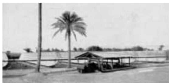
**Figure 3 First parabolic trough plant in Egypt (Source: Stinnesbeck, 1914)<sup>11</sup>**
