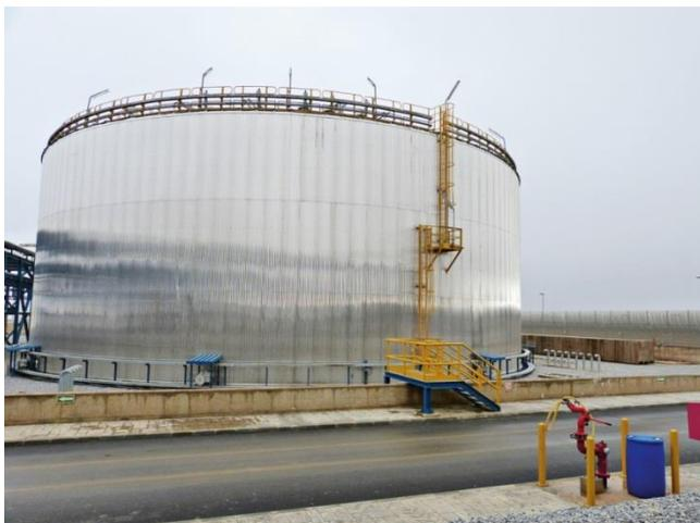
Fig. 4: One tank of a two tanks molten salt system in a solar thermal power plant.
