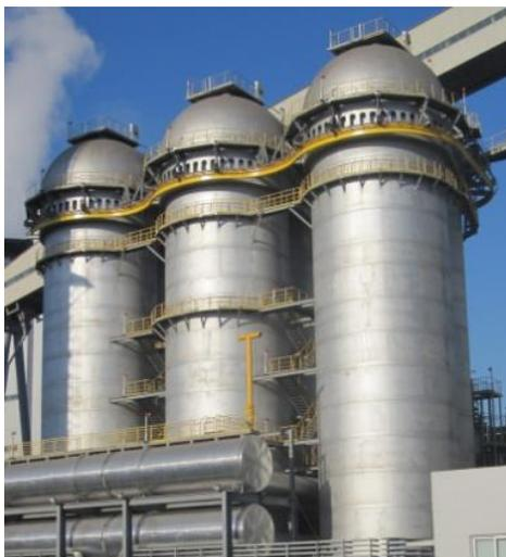
Fig. 2: Photo of a regenerator (or Cowper) for sensible heat storage in solids (Source: Paul Wurth).
